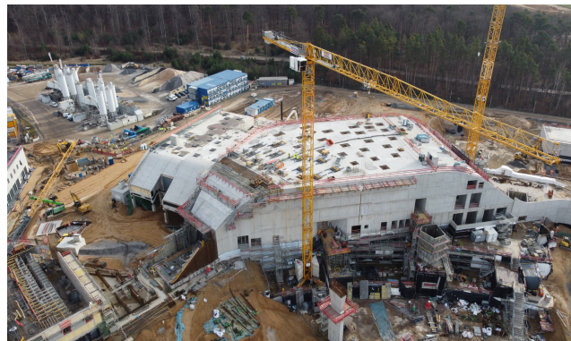
construction area south
