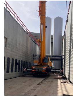
Apr'24 six He tanks of the cryo facility were installed
