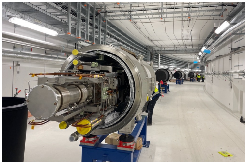
installation of SIS100 dipoles Apr'24
