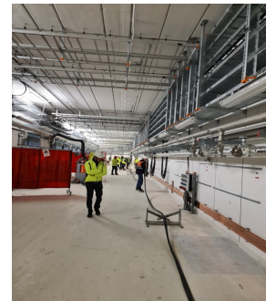
start of cable pulling work, Q3/23
