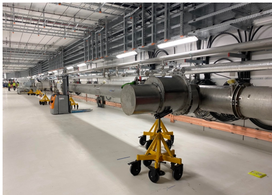
cryogenic bypass lines placed in SIS100 tunnel, Apr'24
