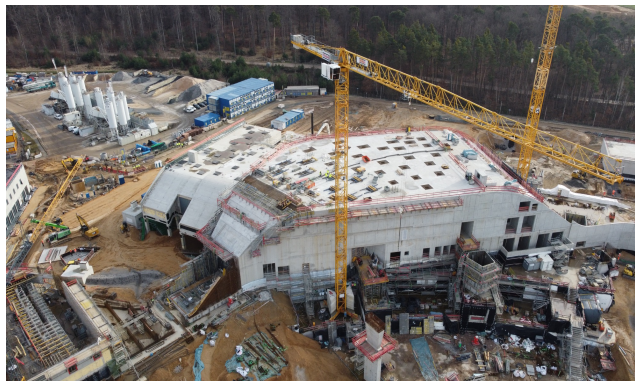
construction area south
